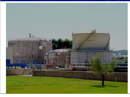
Anaerobic digesters at the bottom of the image, gasholder in front.
