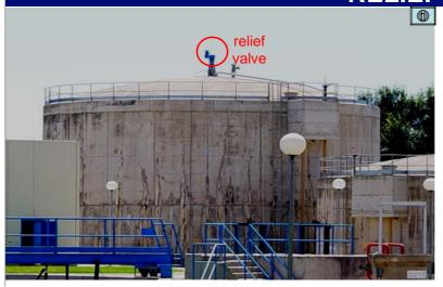
The relief valve on top of the digester prevents an increase of pressure exceeding design values. Some space for the gas is allowed at the top of the dome.
