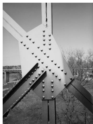
b) https://commons.wikimedia.org/wiki/File:THROUGH_TRUSS_VERTICAL-DIAGONAL_INTERSECTION_DETAIL_-_Richmond_Bridge,_US_90A_at_Brazos_River,_Richmond,_Fort_Bend_County,_TX_HAER_TEX,79-RICH,2-25.tif?uselang=es
