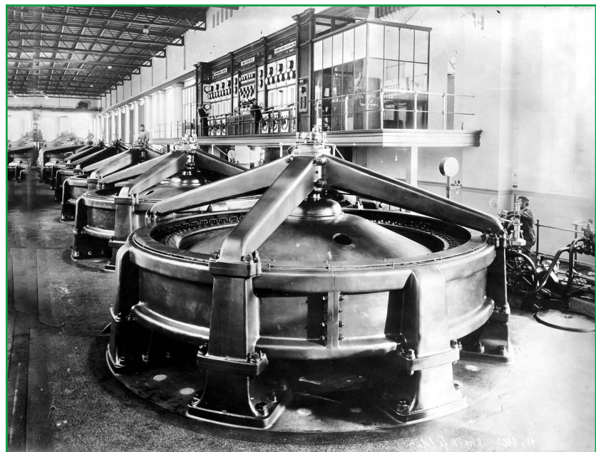
figure 7. Rheinfelden hydroelectric power station on the upper Rhine River, 1898, showing 850-hp, three-phase ac generators having 88 poles and operating at 68.2 rev/min and 50 Hz (photo courtesy of Energiedienst Holding AG Laufenburg).
