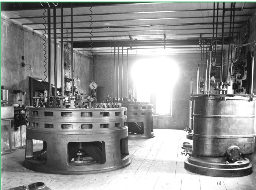
figure 2. Hochfelden hydroelectric power station near Zurich, 1892, showing “Type Lauffen vertical” three-phase ac generators operating at 187.5 rev/min and 50 Hz (photo courtesy of ABB Switzerland).
