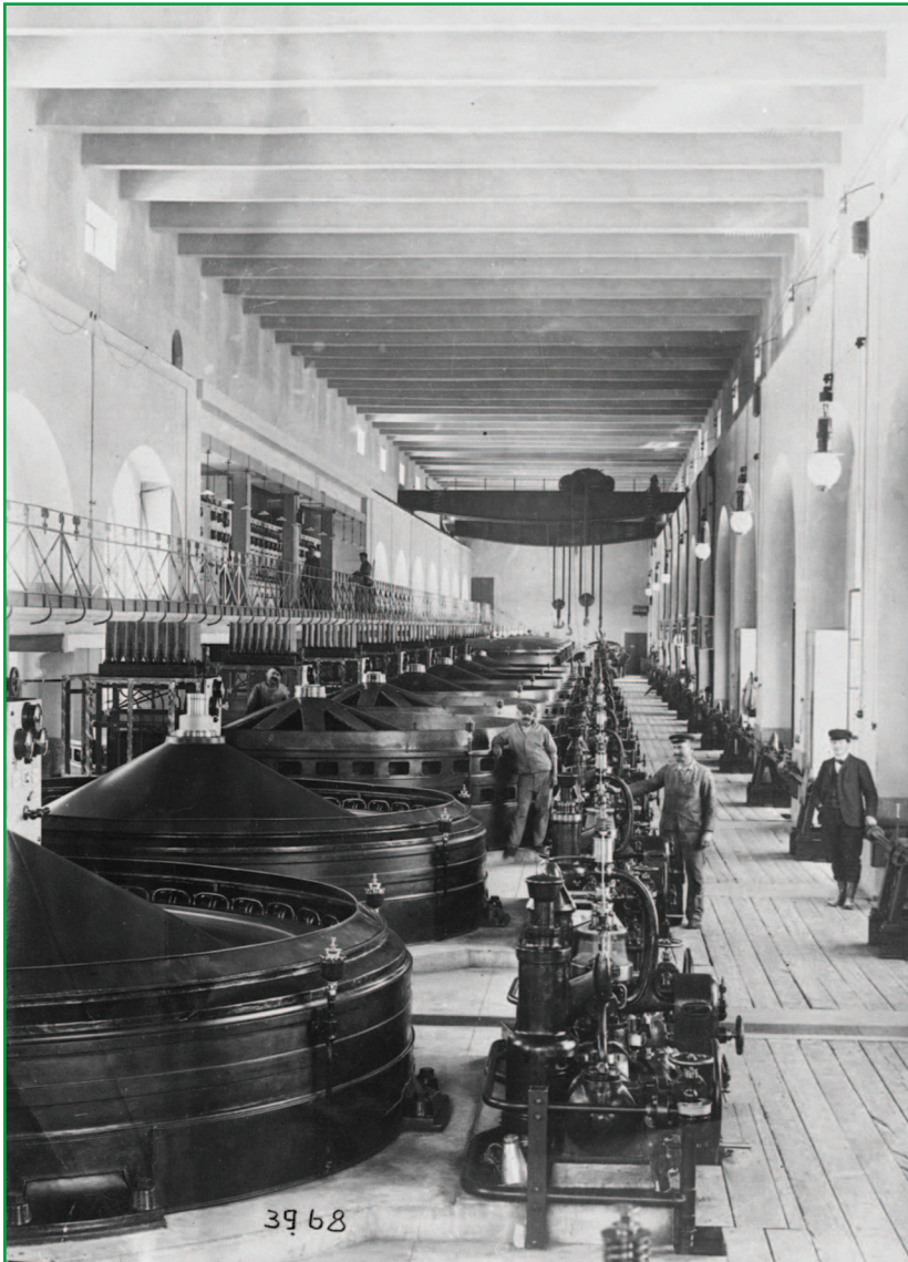
figure 10. Chèvres hydroelectric power station on the Rhone River, around 1900, showing two-phase ac generators having 46 poles and operating at 120 rev/min and 46 Hz, a first delivery lot had another combination of pole numbers and revolutions (photo courtesy of ABB Switzerland).
